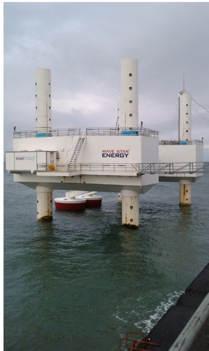
The Roshage test unit and close up of floats
