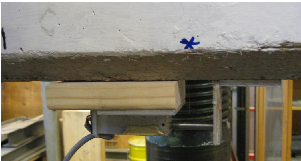
Figure 3. Shown is the LVDT-gauge mounted across the crack.
